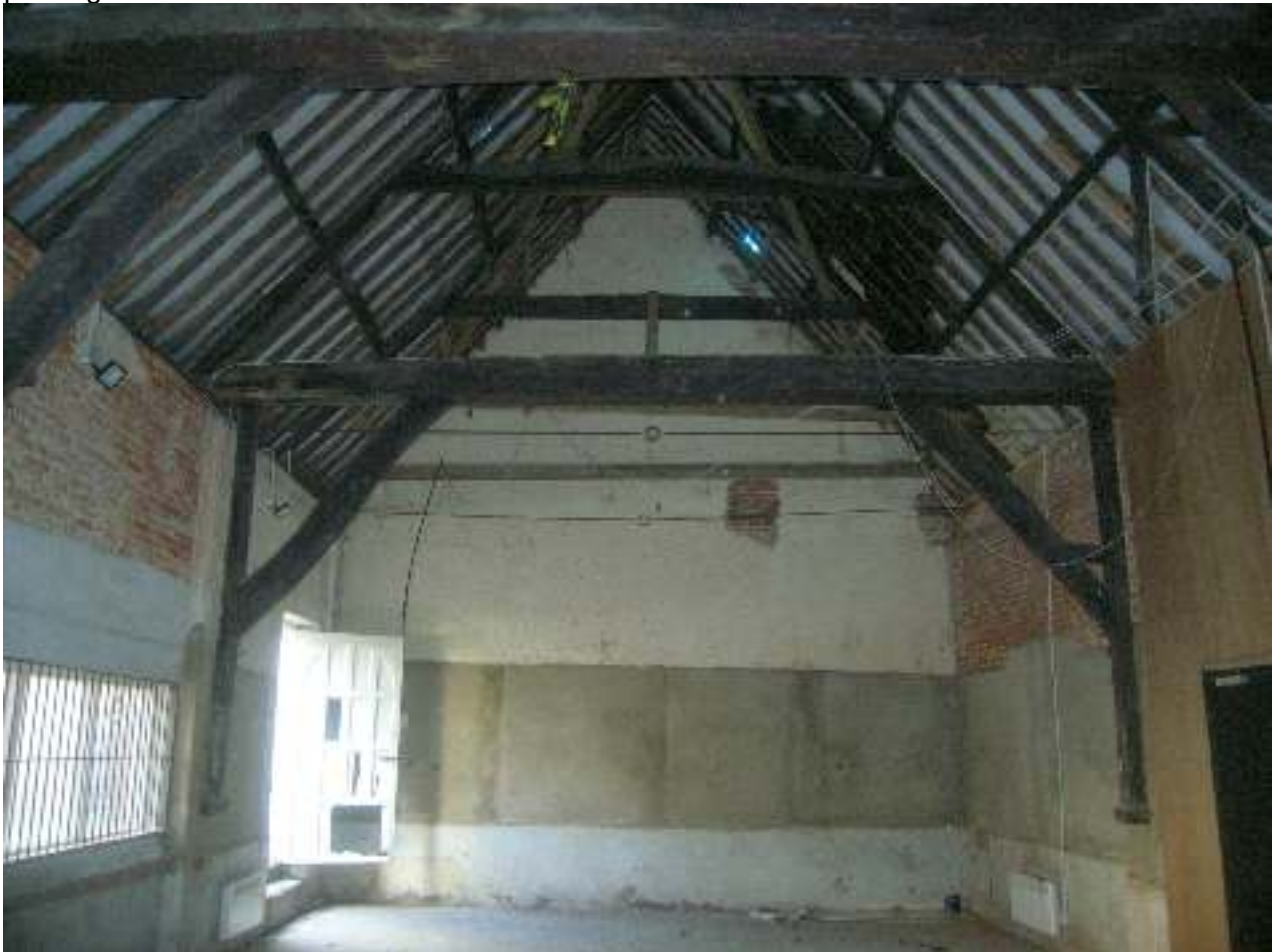
North gable wall and northernmost braced tie beam
