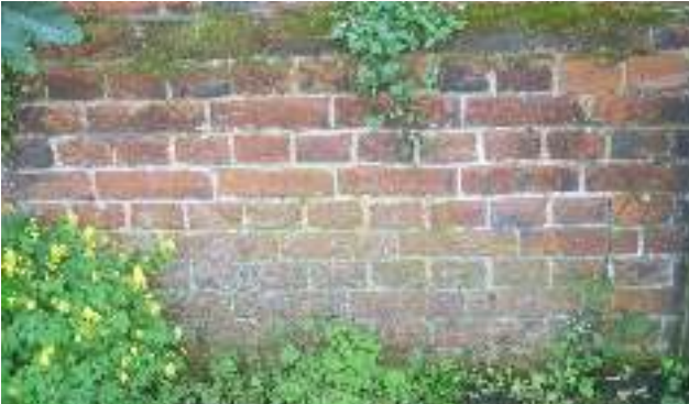
English bonded brickwork to plinth – alternating courses of brick sides (stretchers) and brick ends (headers).
