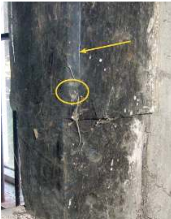
Chamfered edge (arrowed) with run out stop (circled) at bottom
