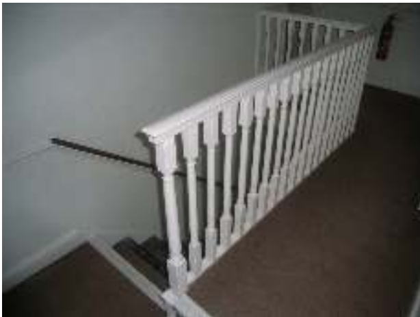
The stairs in the circa 1800 rear wing lead up to a fashionable landing designed into the layout which provides direct access to all first floor rooms.
