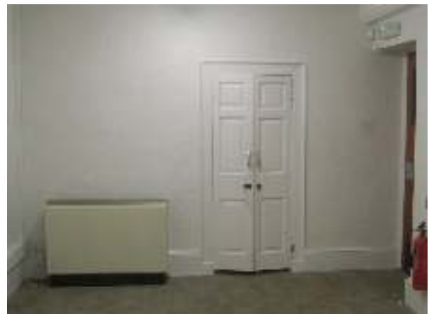
Opposite the windows of the reduced width room, a pair of double doors dating from circa 1800 once led into the southernmost rear wing. The double doors now just open into a deep storage cupboard.
