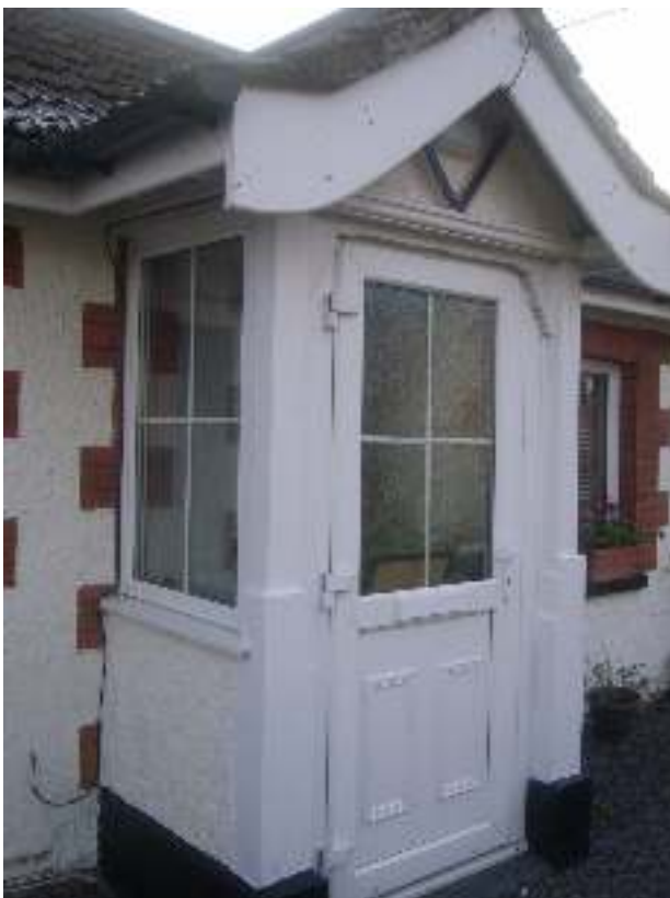
On the porch facing Pound Lane, the art deco detailing half-way up the sturdy timber posts forming the front corners, intricate scrolling to the head board over the door, and the way the side walls and windows randomly cut across the red brick quoins of the main wall, all mark it out as originally an open-sided, open-fronted porch probably added around 1930.
